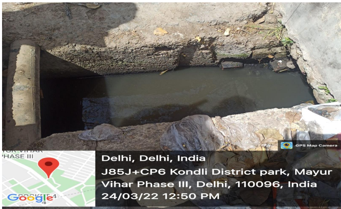
Figure 2: Diversion at Kondli
